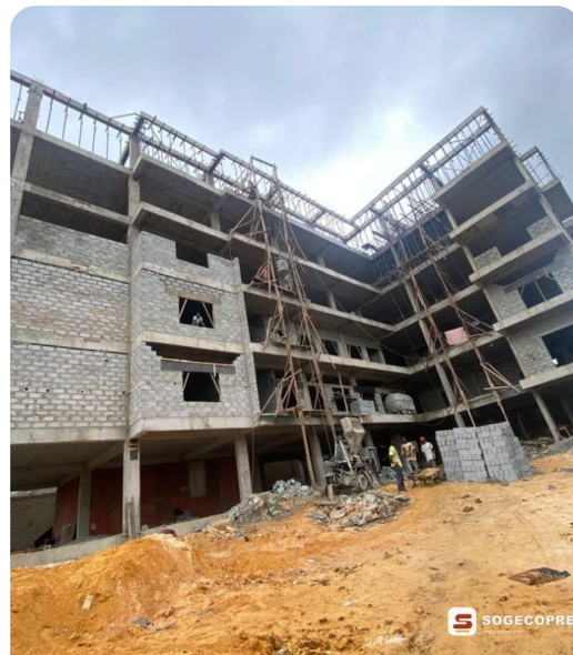
Private building in Kipé — SOGECOPRES site
